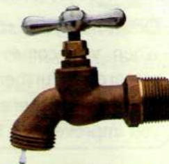
tap is leaking
